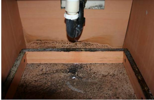
Inspection #1: Leaking J trap caused mold and mildew to form under the sink.
