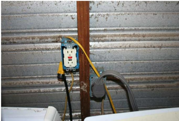
Inspection #13: Lightweight extension cord stretched from the main home to the storage shed to supply power posing a potential electrical hazard.
