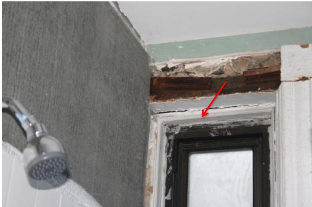
The picture above shows the results of a water leak rotting the wood above the bathroom window.
