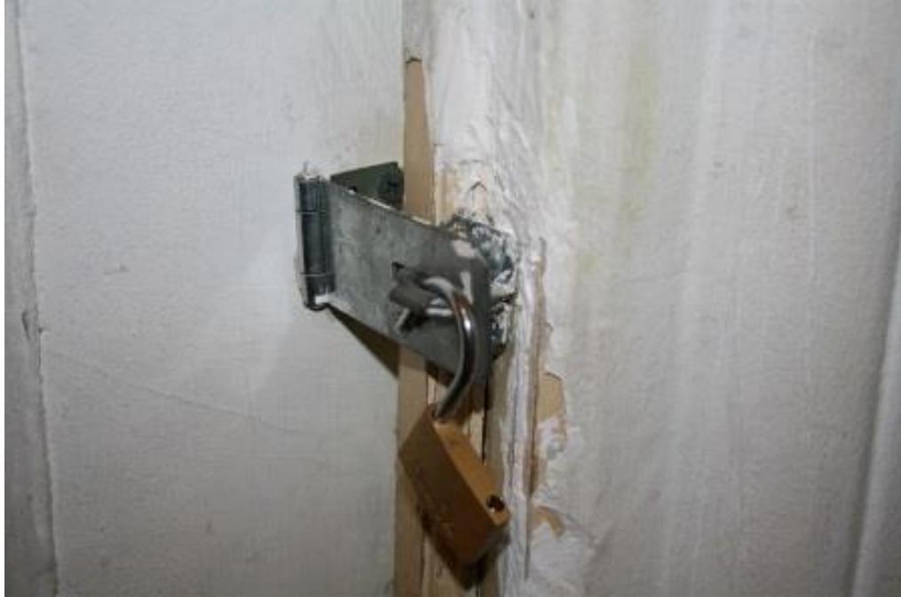
The picture above shows a hasp and lock on the door of the left front bedroom. This type of lock is considered a potential trapping hazard. This unit contained additional violations, such as a smoke detector mounted 27 inches from the ceiling, which was more than the 12-inch requirement, and an unsecured cover on the junction box.
