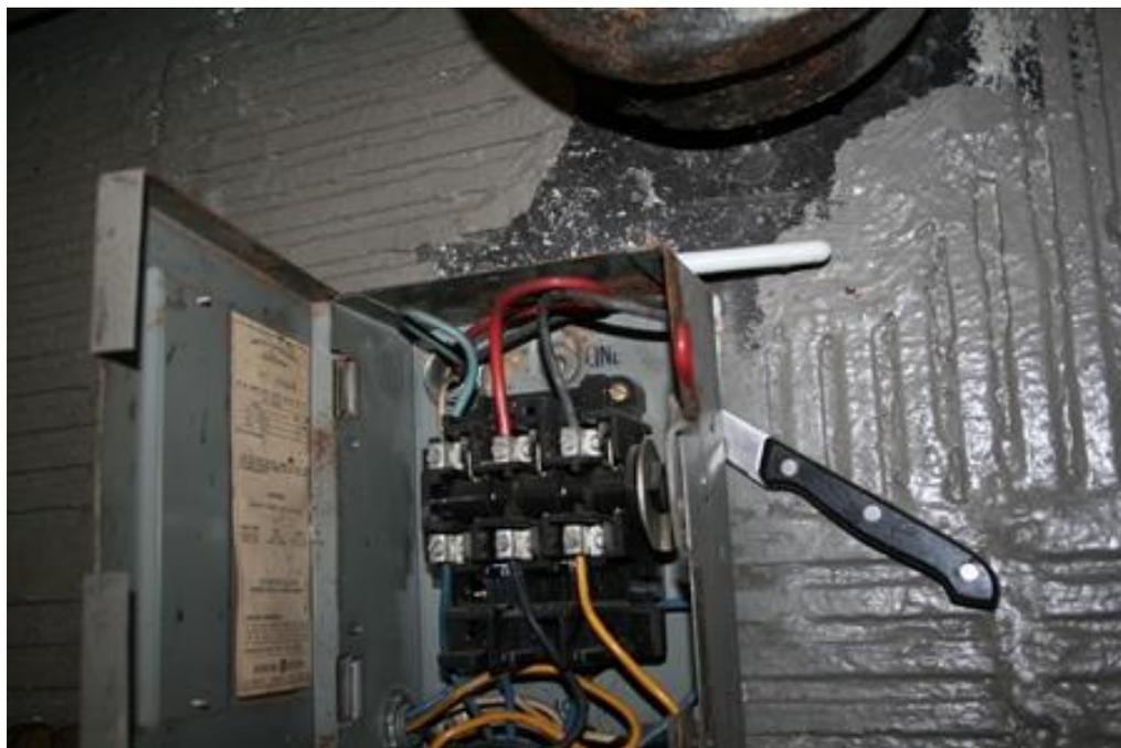
The picture above shows an unsecured cover on a disconnect box with exposed wiring and contacts in the building basement garbage room. The laundry room for tenants was located in the basement.
