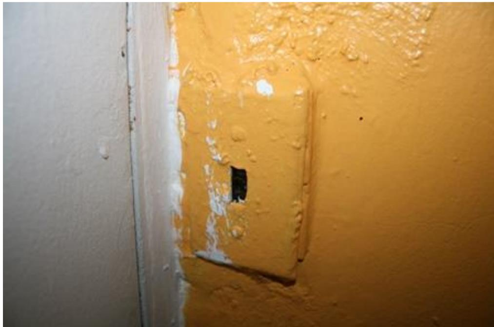
The picture above shows a broken light switch by the entrance to the unit with exposed contacts in the box. According to the tenant, this switch had been broken for at least 6 months. The unit was inspected by the Authority on January 24, 2013, and by our inspector on April 25, 2013.
