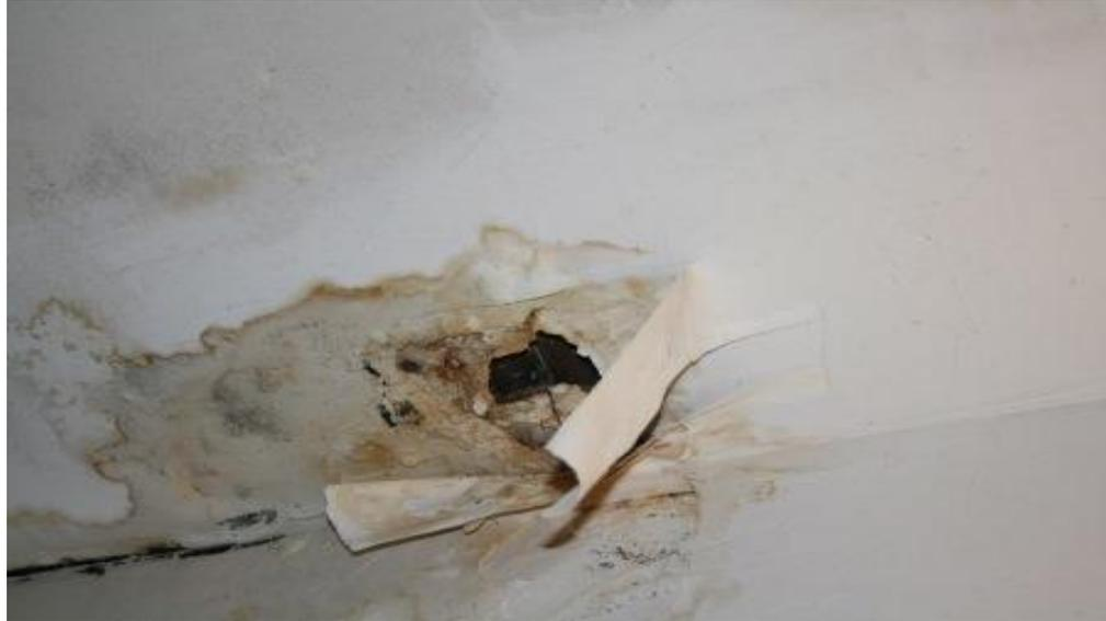
The picture above shows a hole in the unit ceiling above the bathtub. According to the tenant, the hole was patched up by the landlord but continued to leak at times.
