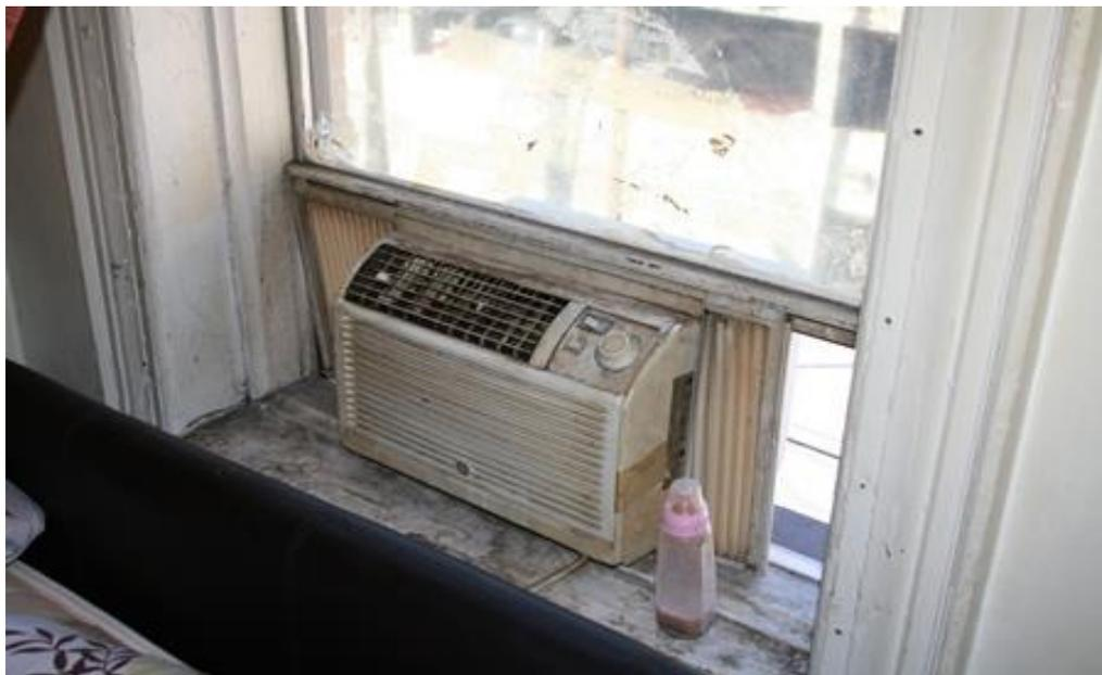
The picture above shows an air conditioning unit not properly secured to the window, which posed a potential falling hazard. Also, there was an open space between the air conditioning unit and the window frame, which presented a falling hazard for a child under the age of 6.
