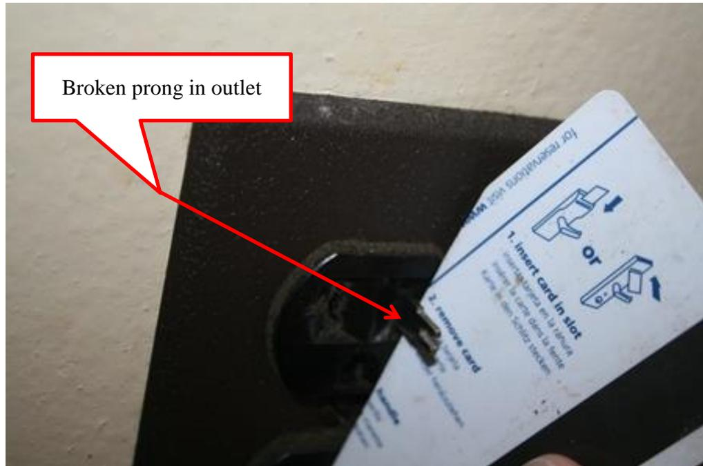
The picture above shows a broken prong sticking out of an outlet in the kitchen. The broken prong had an electrical current.
