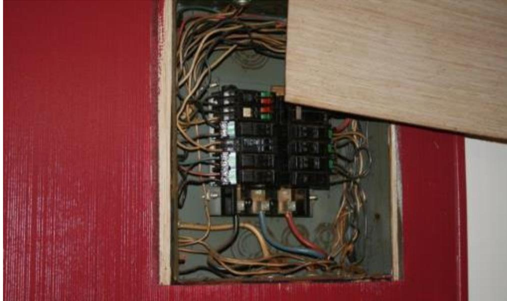
The picture above shows a missing cover on the breaker box panel in the kitchen. A piece of wood was used to cover the exposed wiring in the breaker box, which presented a potential electrical shock hazard. There was also a 2-year-old child residing in the house.
