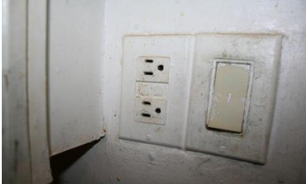
The picture above shows a ground fault circuit interrupter in the bathroom, which did not trip because it was painted over. This unit contained additional violations, such as a light fixture hanging from the wires and not properly secured to the ceiling; excessive grease on the kitchen stove, walls, and cabinets; overcircuited outlets; and a rear window that would not stay up.
