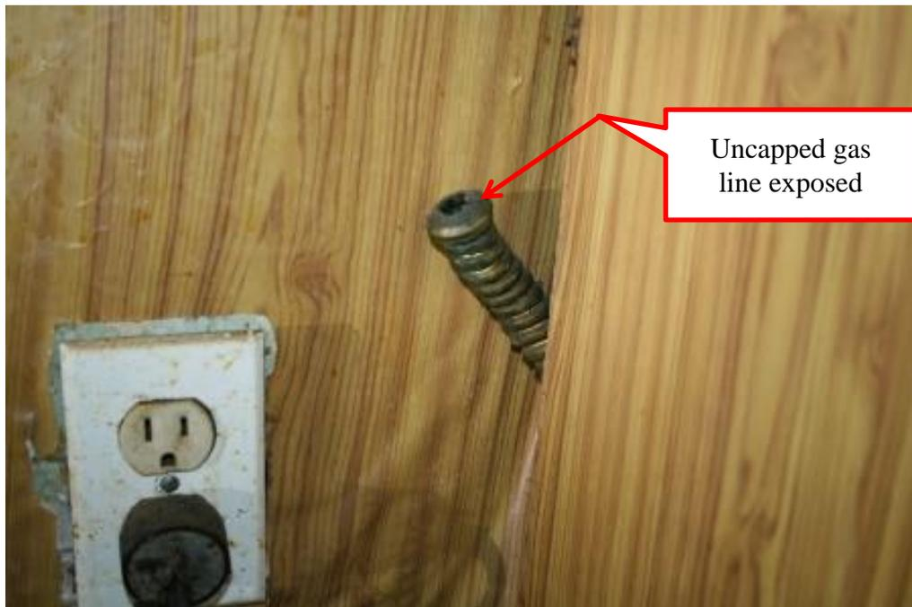
The picture above shows an exposed, uncapped gas line in the kitchen next to an electrical outlet. This is considered a fire hazard.
