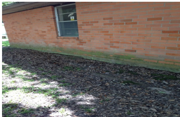
Illustration 1: Unit buildings with mud and mildew buildup on lower bricks
