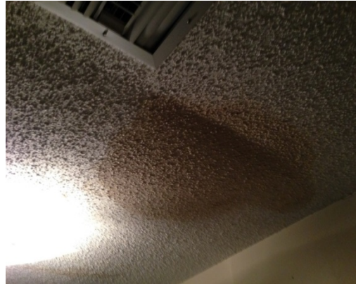
Units with peeling paint and stains on the ceiling
