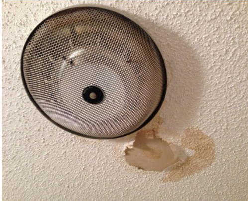
Units with peeling paint and stains on the ceiling
