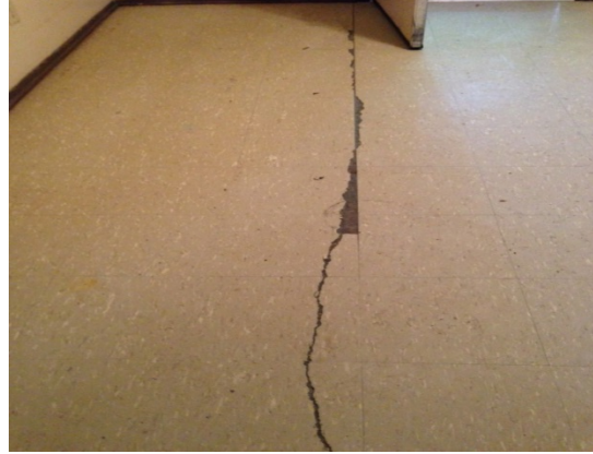
Units with cracked or missing floor tiles
