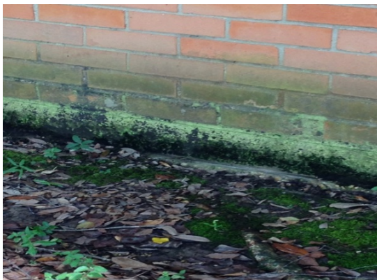
Illustration 1: Unit buildings with mud and mildew buildup on lower bricks
