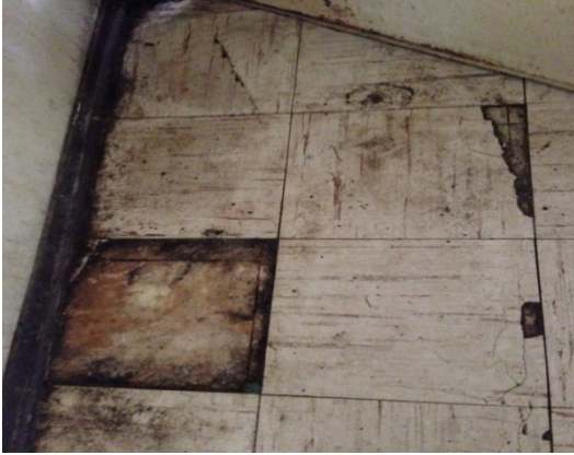
Units with cracked or missing floor tiles
