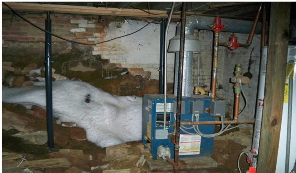
Collapsed foundation wall with snow and mud in the basement
