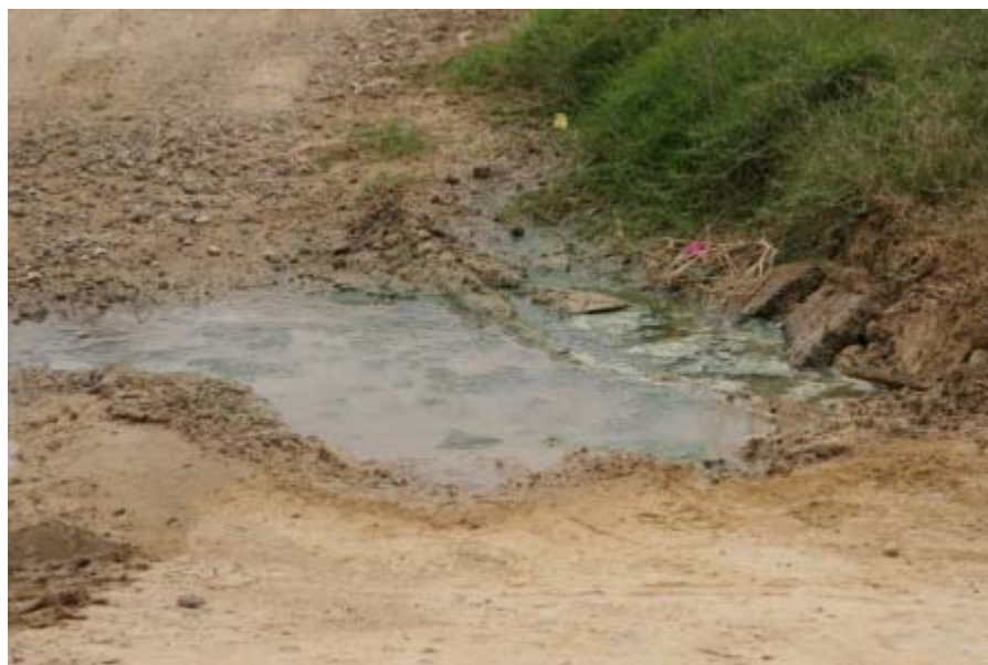
This residence in Tanquecitos 2 Colonia, Webb County, Texas, had wastewater on the unpaved drive to the residence.
