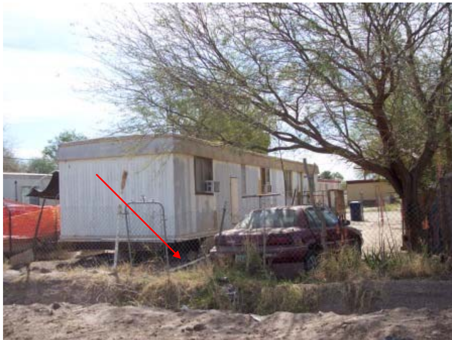
This residence in Drysdale Colonia, Yuma County, Arizona, lacked adequate water and sewage services. Note the waste water line that runs into the open ditch.
