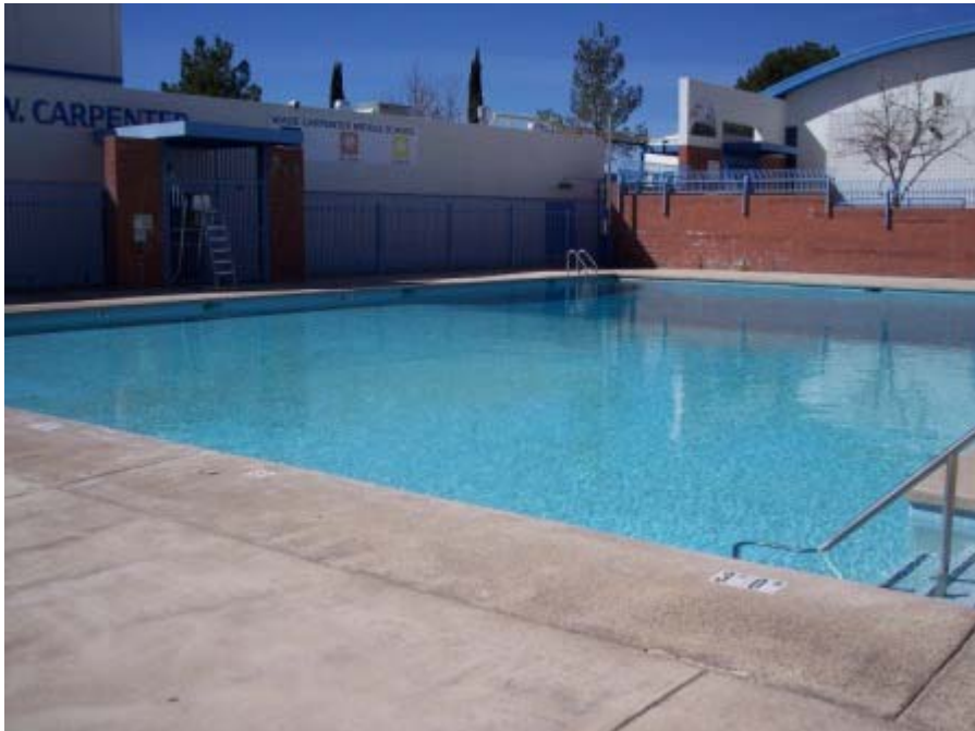
City of Nogales, Santa Cruz County, Arizona, pool improvement.
