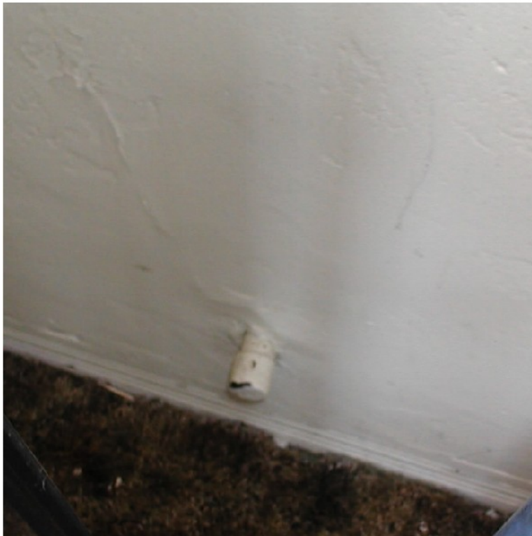
A plumbing pipe was left protruding from a bedroom wall.
