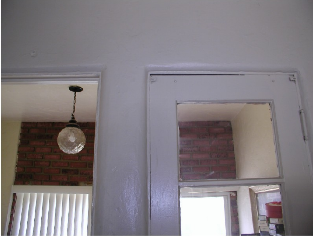
One side of French door to sunroom was painted shut (the other side was operable).
