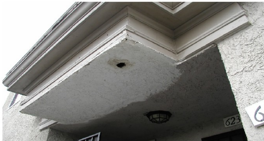
Rainwater downspout was not installed to deflect runoff from the front porch (hazard).
