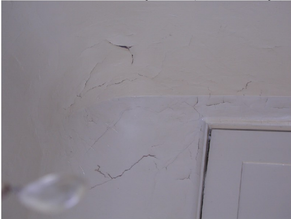
Extensive peeling paint was observed throughout the house. The homeowner stated that this condition occurred within one year after work completion, but when she tried to contact the contractor, he had moved out of state.
