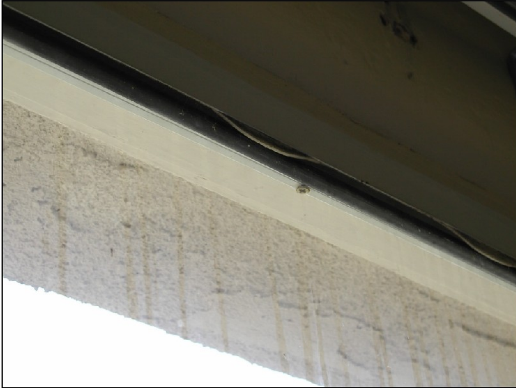
A front living room window (manufactured) was defective and leaked.
