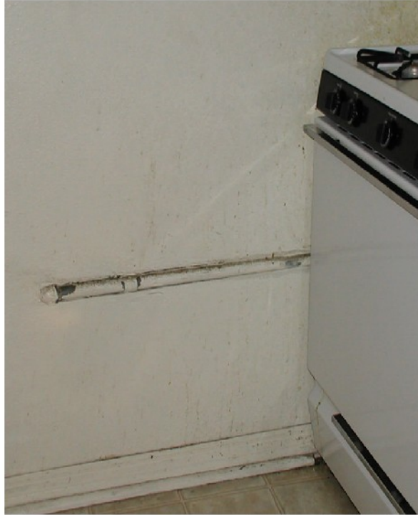
There was an exposed gas line in the kitchen.
