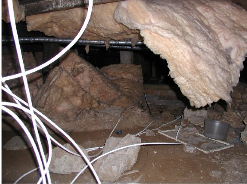
Floor insulation was falling down in the crawlspace due to deficient installation work.
