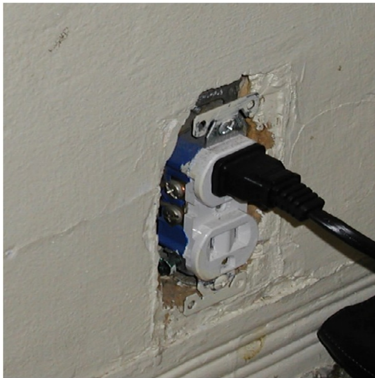
The owner reported that this outlet cover was never installed in the bedroom.
