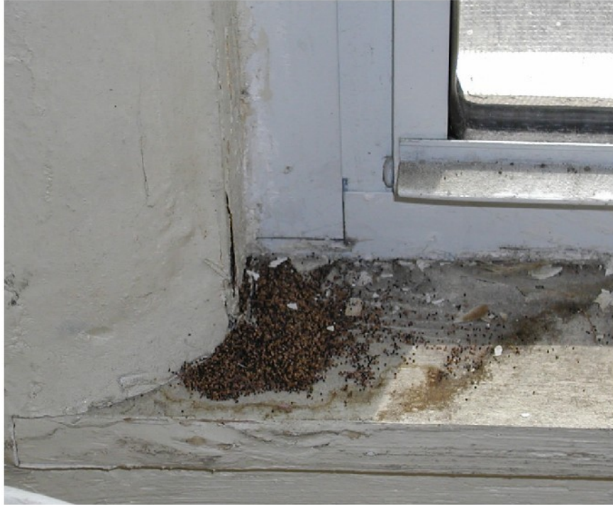
There was wood debris from an active infestation in the bedroom.
