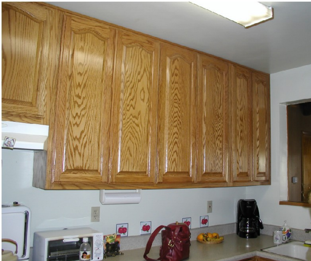
New outlets were installed on an existing laundry circuit, causing the circuit breaker to trip repeatedly (code violation).
