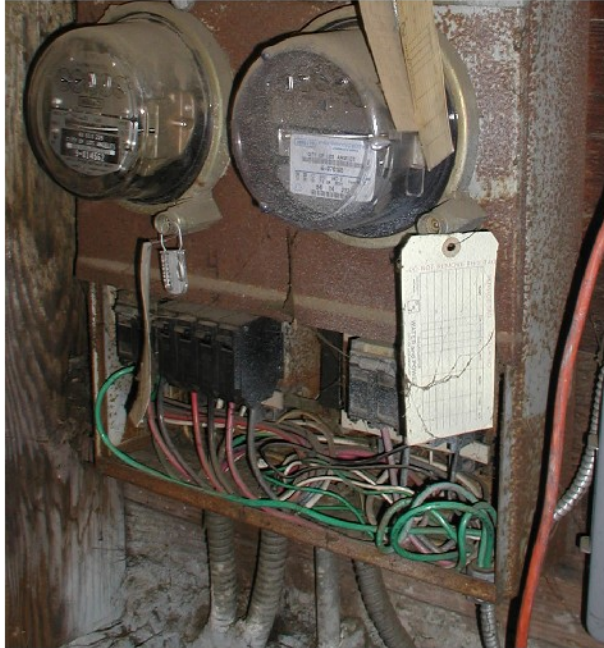
There were exposed wires in the electrical panel.
