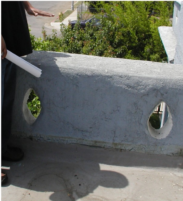
The second story balcony railing was too low, a hazard that was not addressed.
