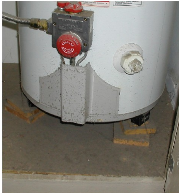
All four units had new interior water heaters installed without the required metal pan for leaks. The inspectors explained that this was a hazard, particularly on the second floor units, because leaks could cause the wood platform to rot and fail under the weight of the appliance.
