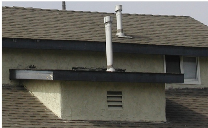
Flashing was not installed where the roof meets the house.
