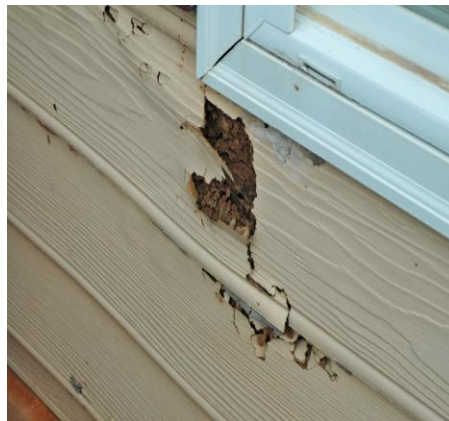
Deterioration caused by boring insects
