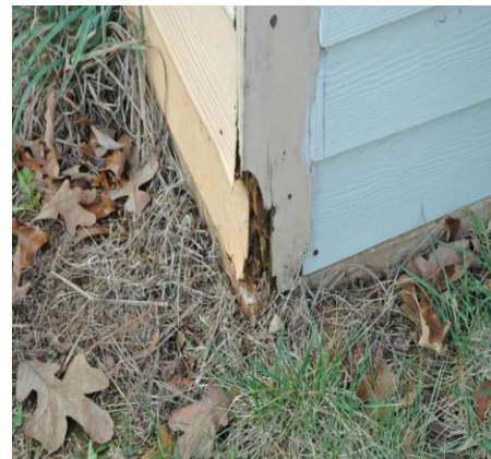
Deterioration caused by boring insects
