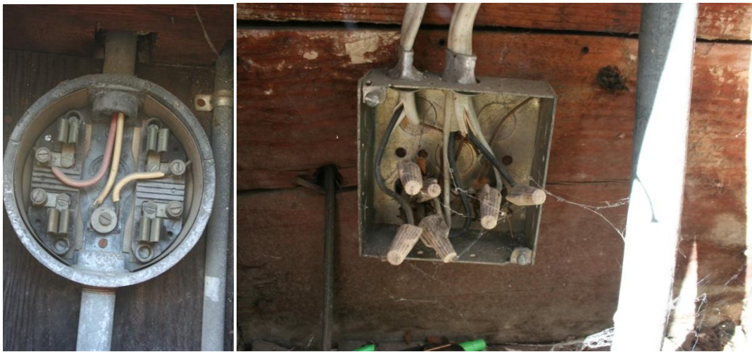
Left – exposed electric meter; right – exposed wiring without a face plate
