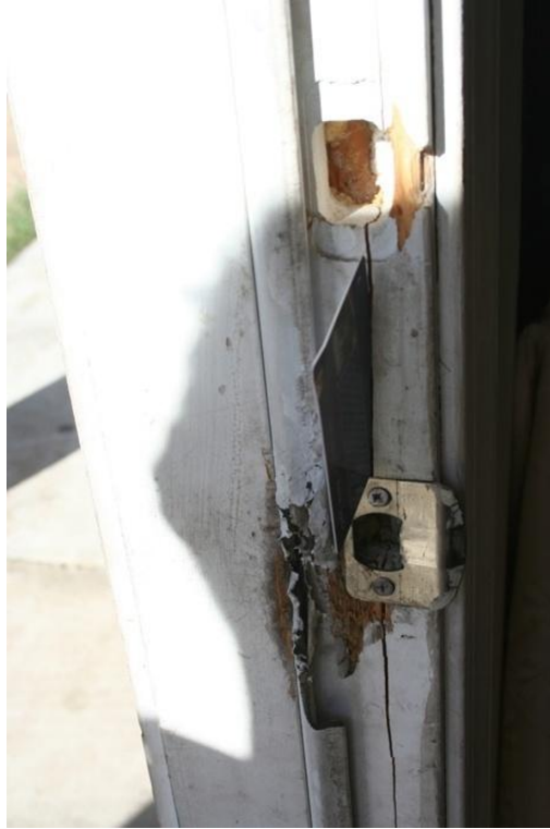
Door frame split and deadbolt missing striker
