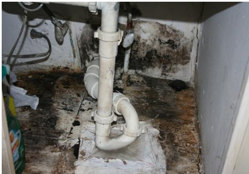
Moisture from continuous leak caused wood rot, holes, and mold/mildew in and around the sink area
