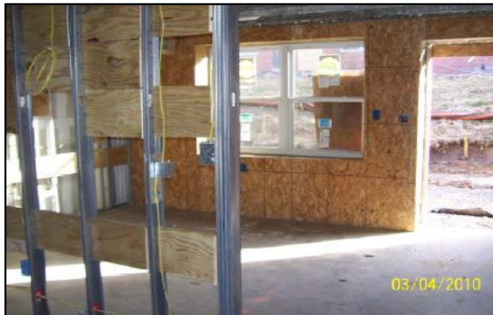
Rehabilitation of units at Howard Day Homes (ongoing)
