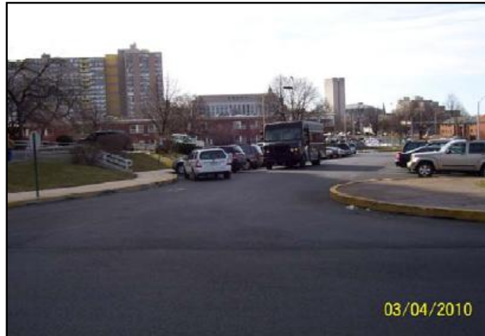
Repaving of parking lot at Lick Towers (completed)
