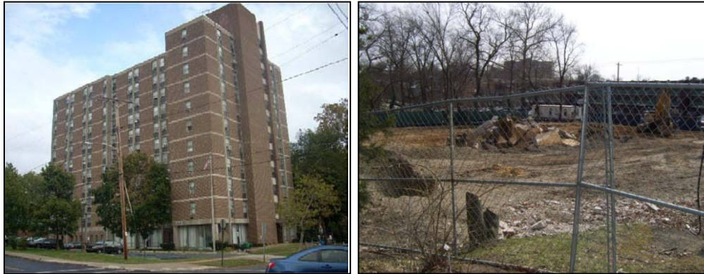
Before (left) and after (right) pictures illustrate the demolition and redevelopment of Lincoln Towers (ongoing).
